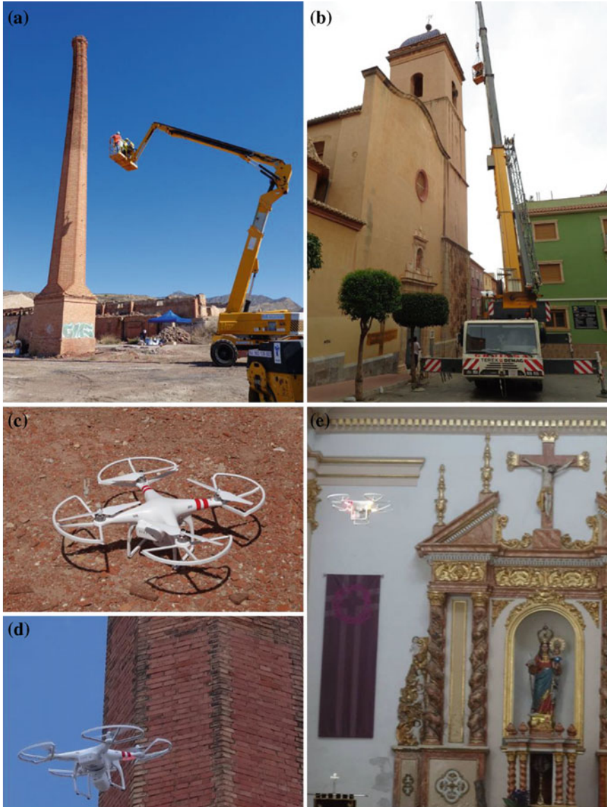
Fig. 2 Human visual inspection: a masonry chimney and b bell tower, both protected structures in Agost (Alicante). c UAV for automated inspection used in d masonry chimney and e interior inspection of Saint Peter’s Church, both in Agost
