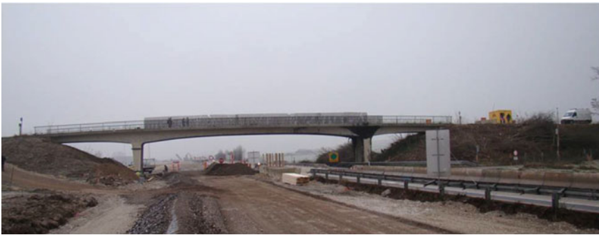
Fig. 6 Bridge S101 during damage test [23]
