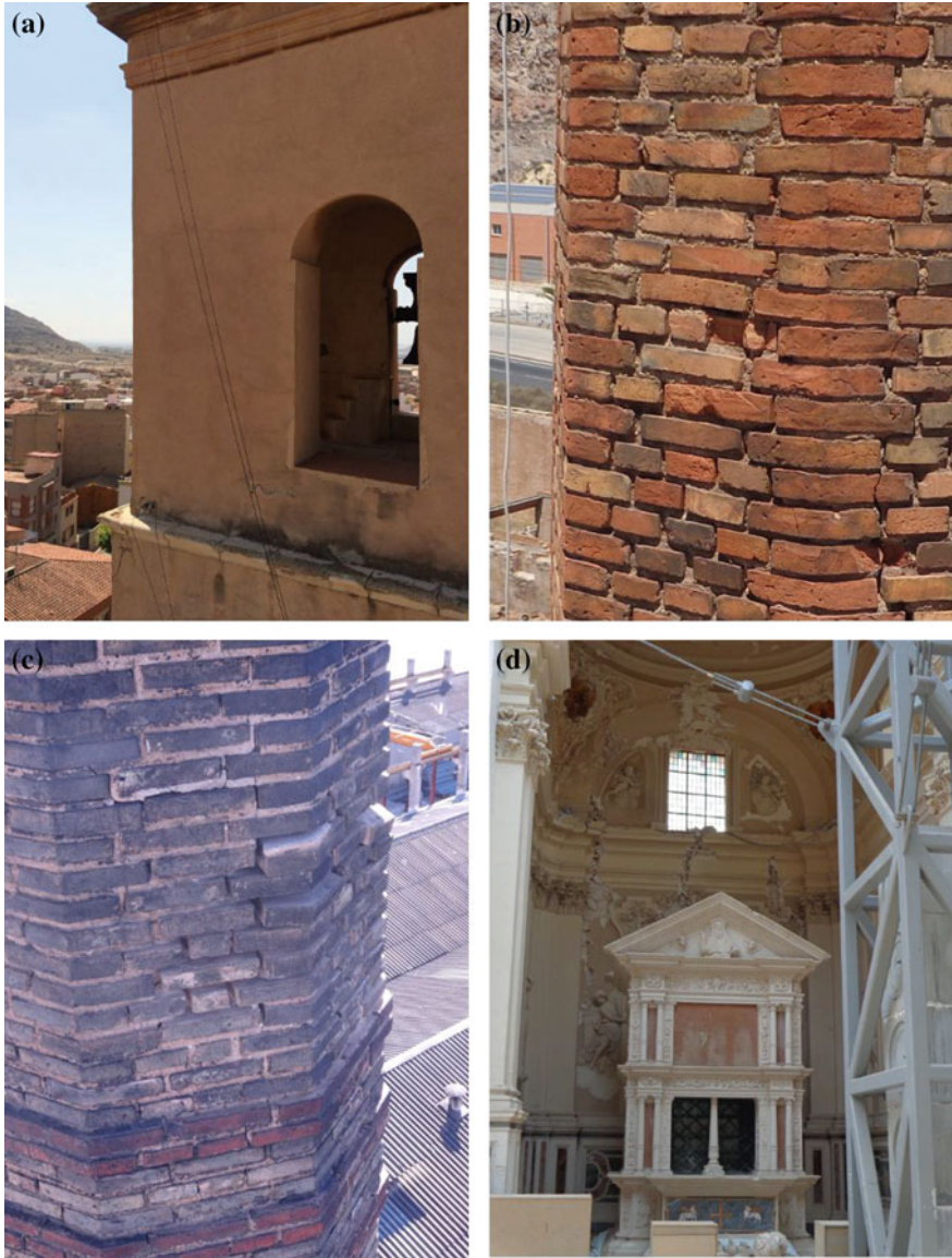
Fig. 1 The most frequently observed pathologies in built heritage: a discoloration, b spalling, c mortar loss, d cracking
