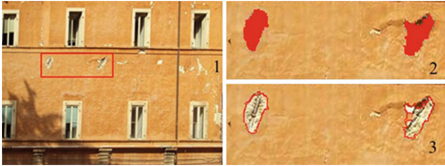
Fig. 6 Example of defect analysis by DIP: from the original image (1), the crop area (2) is selected identifying the defect and the boundaries (3)
